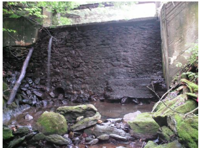
Thunder Brook dam will be removed.
