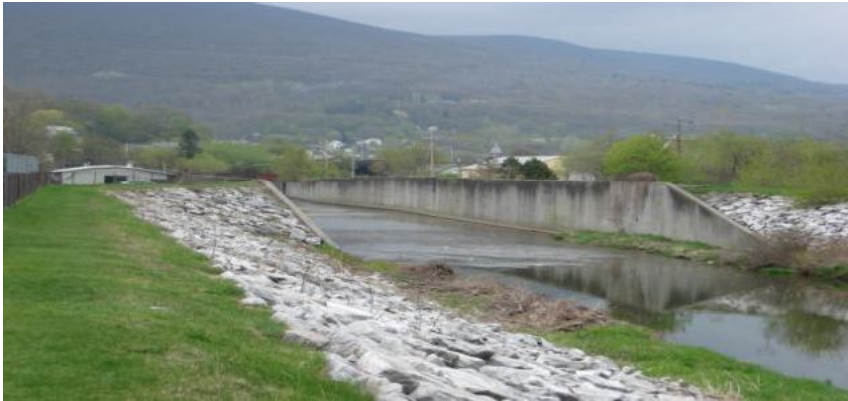
Flood chutes in North Adams.
